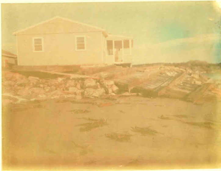
9th St. off E. Grande wooden seawall cement block & slab steps completely gone. 2/7/78
